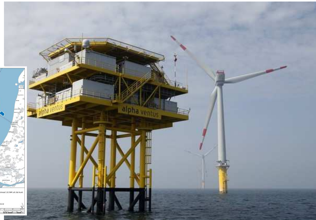
Wind farm transformer station
